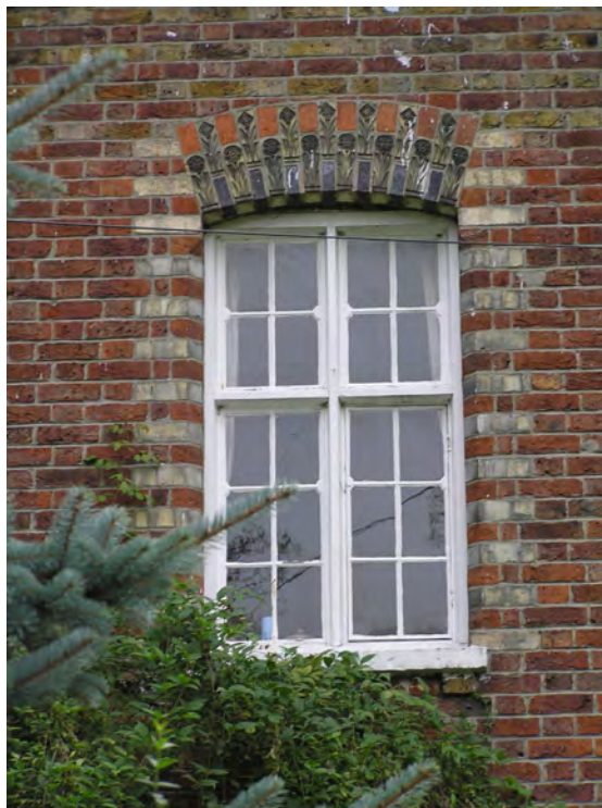
Picture 3.4 Original window detail to Pinnerwood Farm, Woodhall Gate
