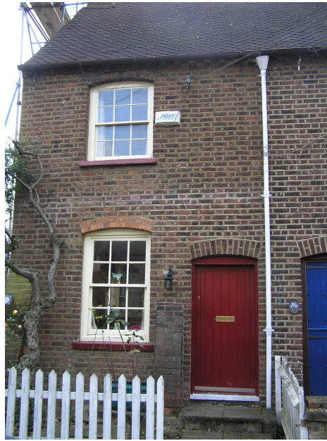
Picture 3.5 29 Middle Road, Harrow on the Hill
