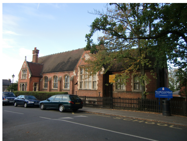
Picture 2.3 John Lyon School, Middle Road, Harrow on the Hill
