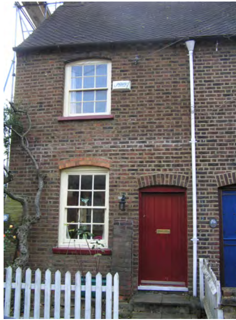
Picture 3.5 29 Middle Road, Harrow on the Hill
