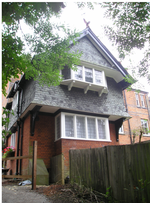
Picture 3.2 Traditional materials and methods to Orchard Cottage, Harrow Park, Harrow on the Hill
