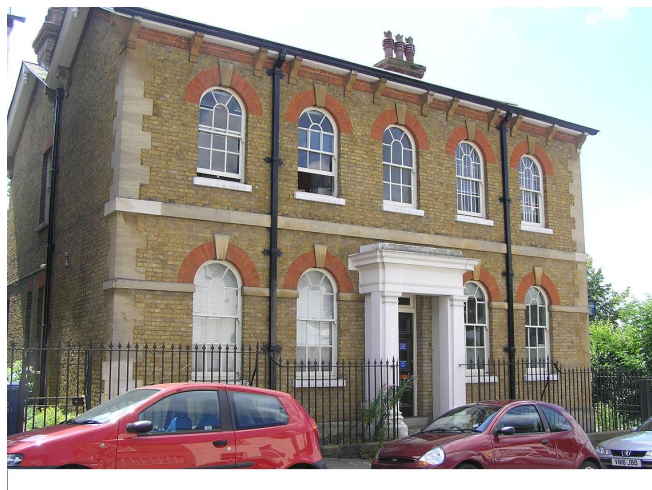
Picture 1.1 Former Police Station, West Street, Harrow on the Hill
